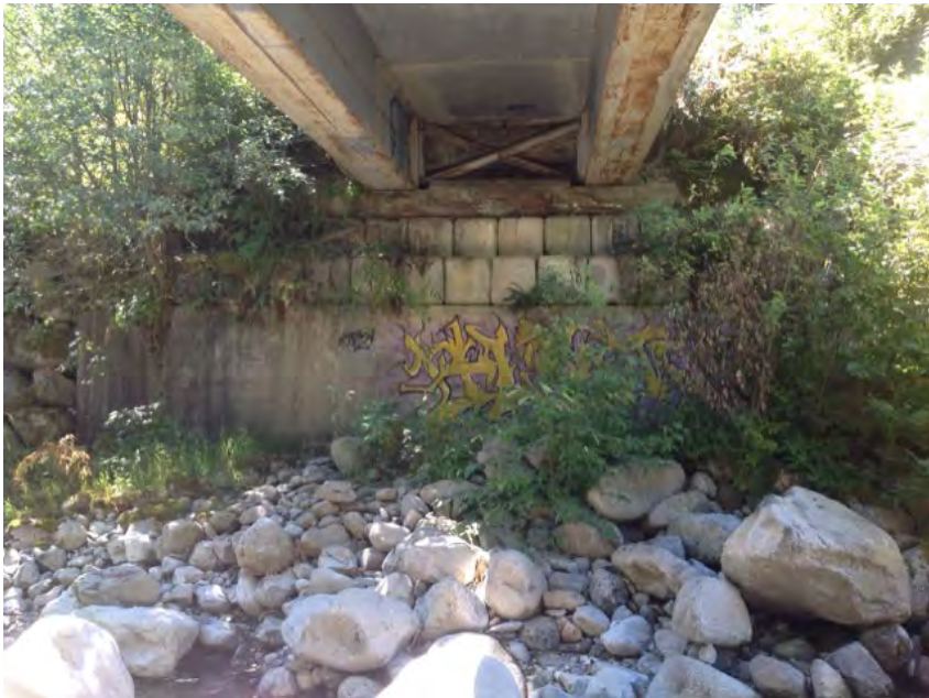
Right Bank Abutment when facing downstream
