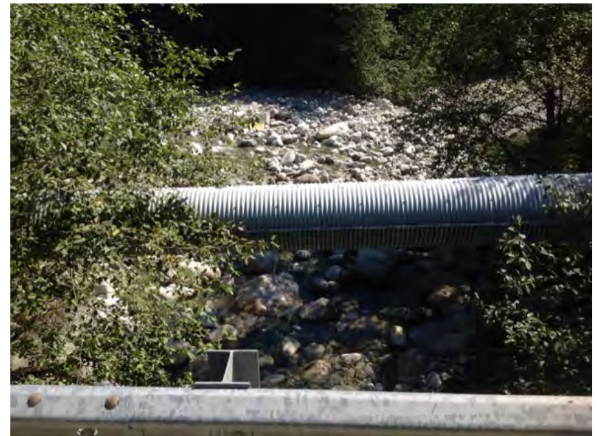
looking downstream from deck
