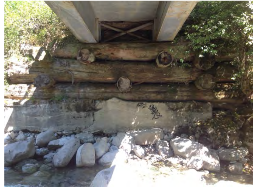
Left Bank Abutment when facing downstream
