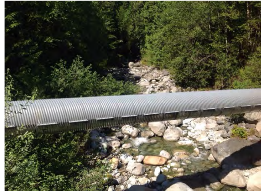
looking upstream from deck
